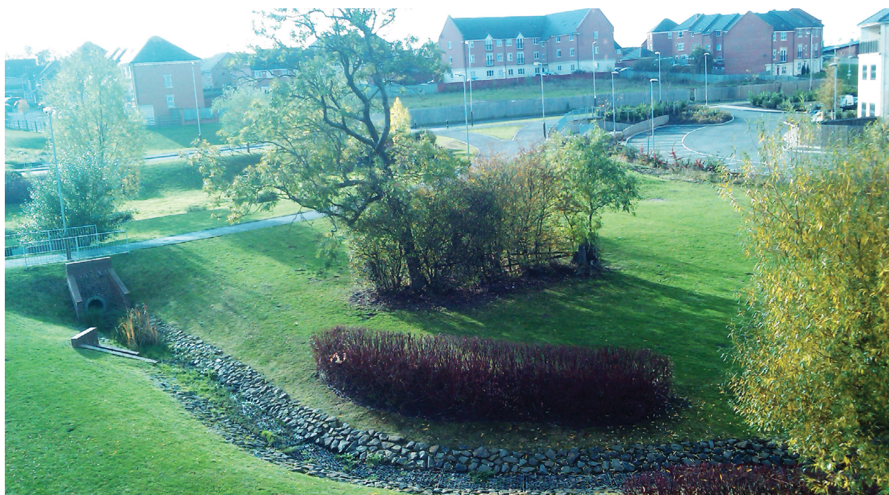
There is growing interest in the East Midlands in using 'natural interventions' to help reduce climate risk (sustainable drainage scheme in Leicester)
